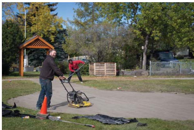
Installation of limestone crush base. October 2016
