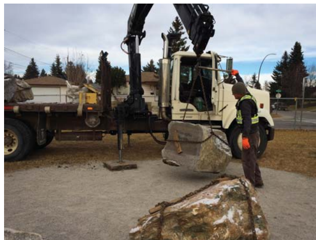
Boulder installation. November 2016
